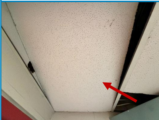
Photo 3: Typical view of the non-asbestos-containing 2'x4 textured pinholes acoustic ceiling tile (see arrow) observed in Corridor near Electrical Room 122 (Loc# 54465).
