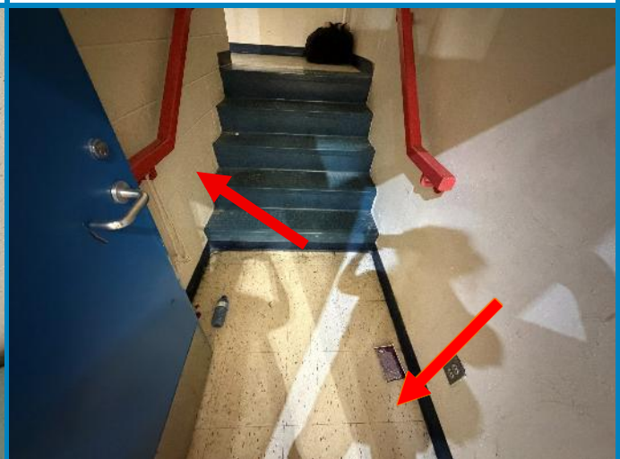
Photo 4: View of the non-asbestos containing 12"x12" white with red, blue, and yellow specks vinyl floor tiles (see right arrow) and non-asbestos containing concrete block mortar (see left arrow) observed within the stair of the stage (Loc# 54529) of the project work area.
