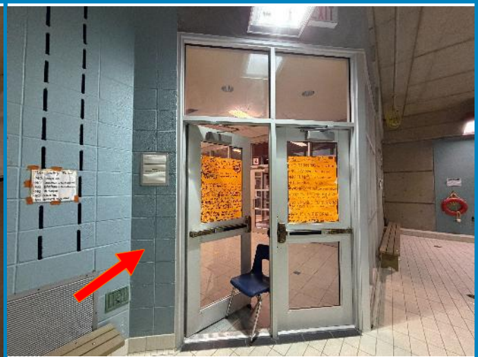
Photo 2: View of the non asbestos-containing blue/white paint compound/sealant (see arrow) observed on the concrete block walls within the Swimming Pool (Loc# 54477).
