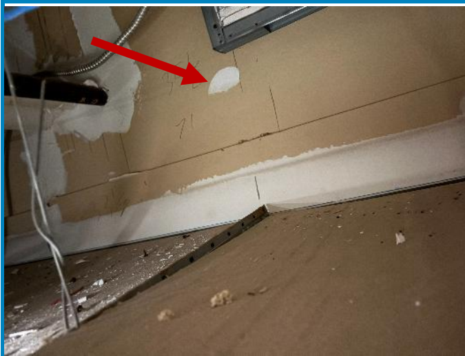
Photo 1: Partial view above ceiling showing drywall wall with non asbestos-containing joint compound (see arrow) that was observed within project work areas.
